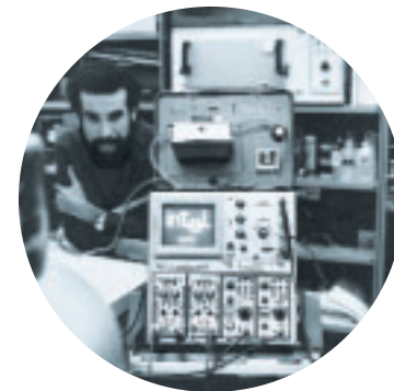
Dov Frohman, inventor of the EPROM, poses with the system he rigged up to demonstrate the new memory technology.
